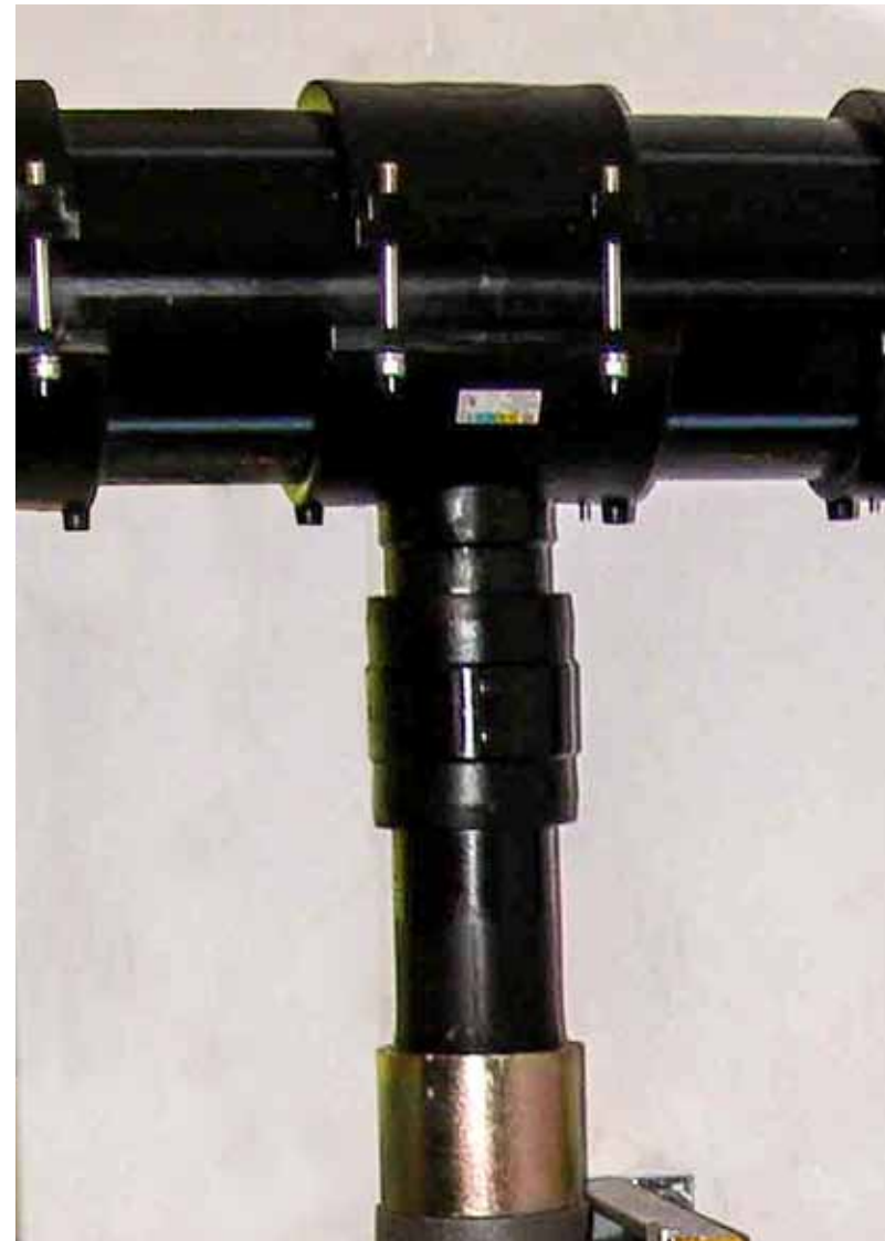
WORK // DRINKING WATER QUALITY IMPROVEMENT PLANT LOCATION // KOVAČIKA
