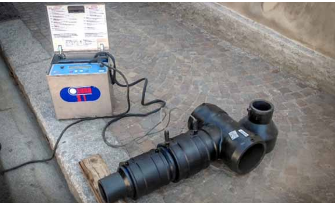
WORK // GAS DISTRIBUTION NETWORK LOCATION // SARDEGNA
