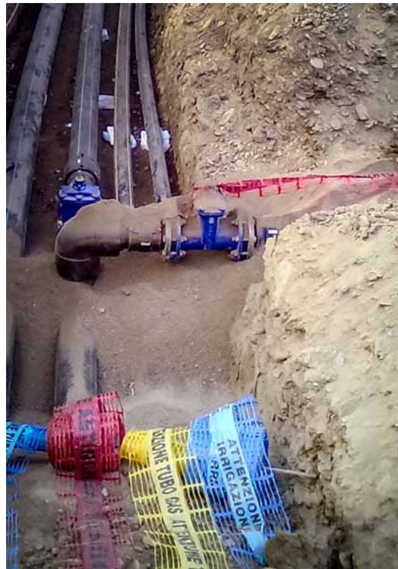
WORK // FIRE-FIGHTING PLANT LOCATION // FIRENZE
