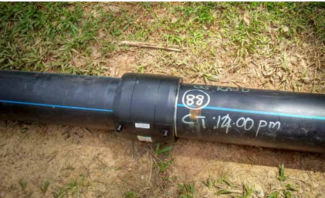
WORK // WATER DISTRIBUTION NETWORK LOCATION // KEDAH
