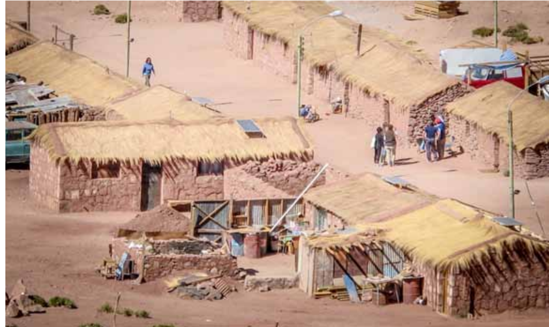
WORK // WATER DISTRIBUTION NETWORK LOCATION // MACHUCA VILLAGE - ATACAMA
