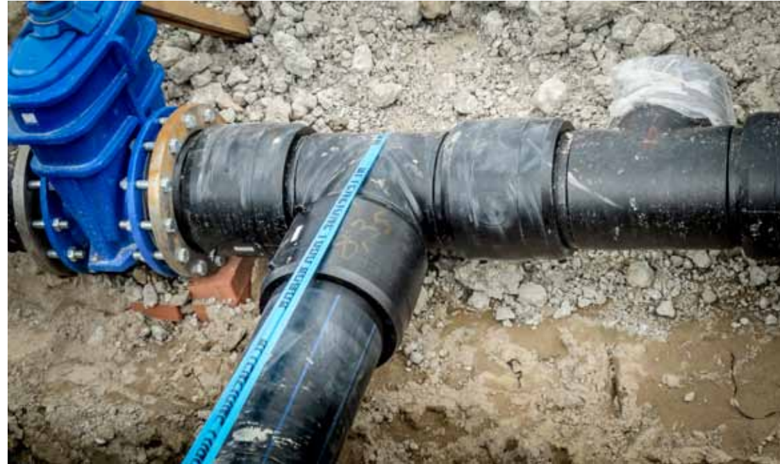
WORK // WATER DISTRIBUTION & FIRE-FIGHTING PLANT LOCATION // PORT - RAVENNA
