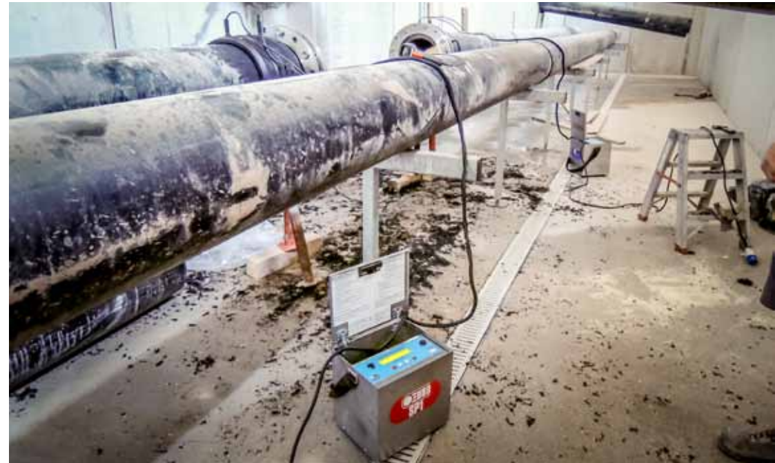
WORK // WASTE WATER TREATMENT PLANT LOCATION // ISCHIA PODETTI - TRENTO
