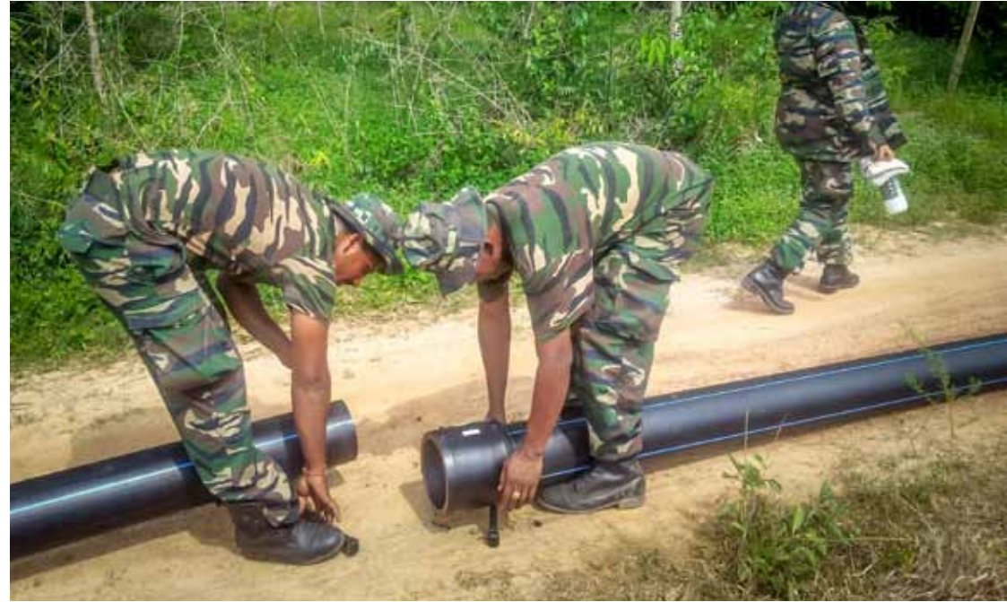
WORK // WATER DISTRIBUTION NETWORK LOCATION // KEDAH
