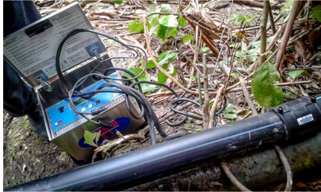
WORK // WATER DISTRIBUTION NETWORK LOCATION // KELANTAN
