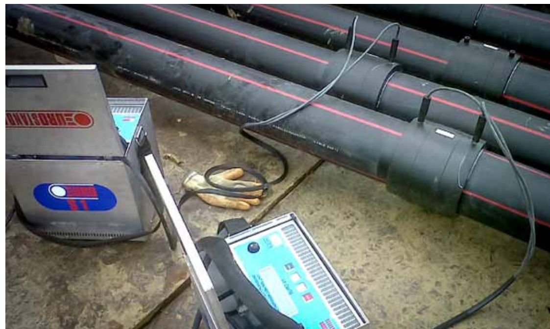
WORK // CABLES PIPELINES LOCATION // CHANCENAY
