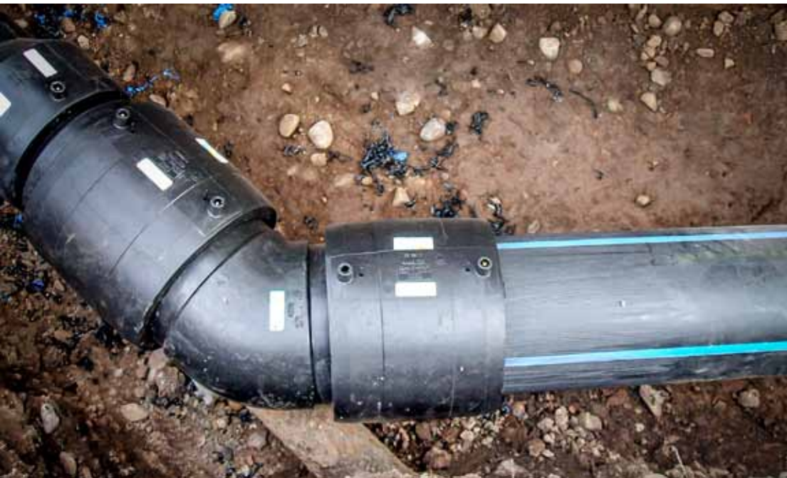
WORK // WATER SUPPLY LOCATION // MEJILLONES
