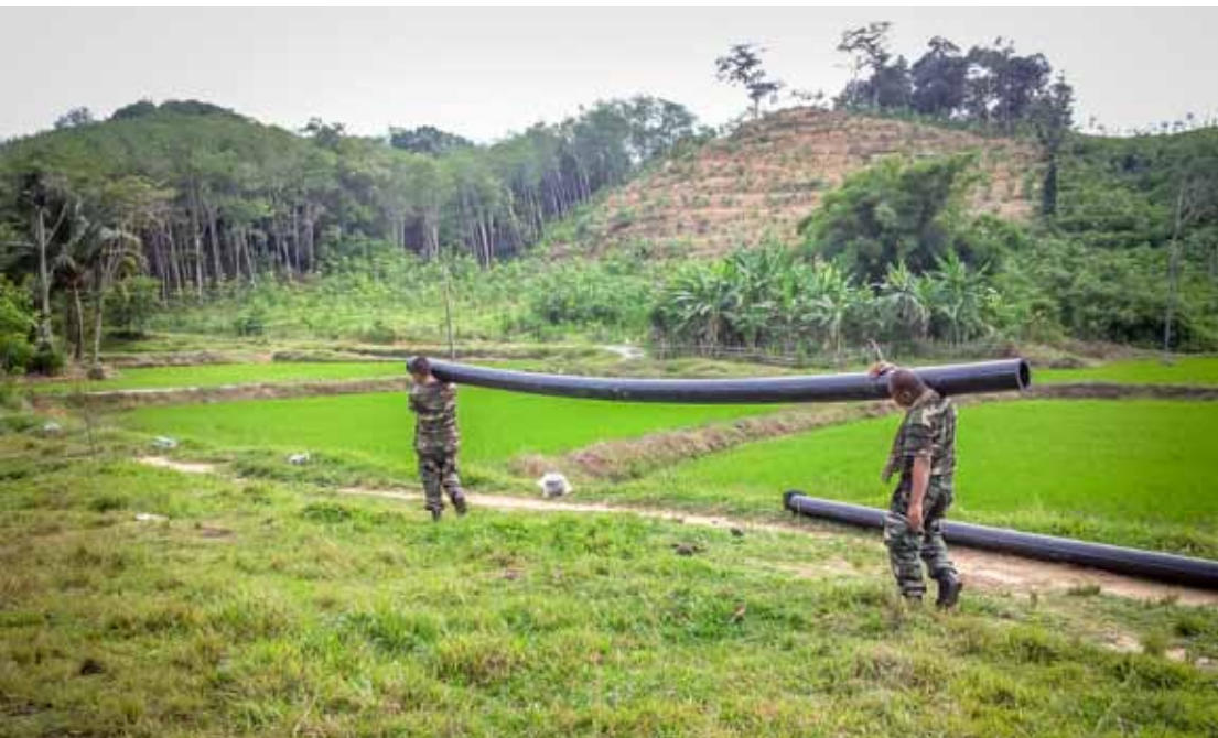
WORK // WATER DISTRIBUTION NETWORK LOCATION // KEDAH
