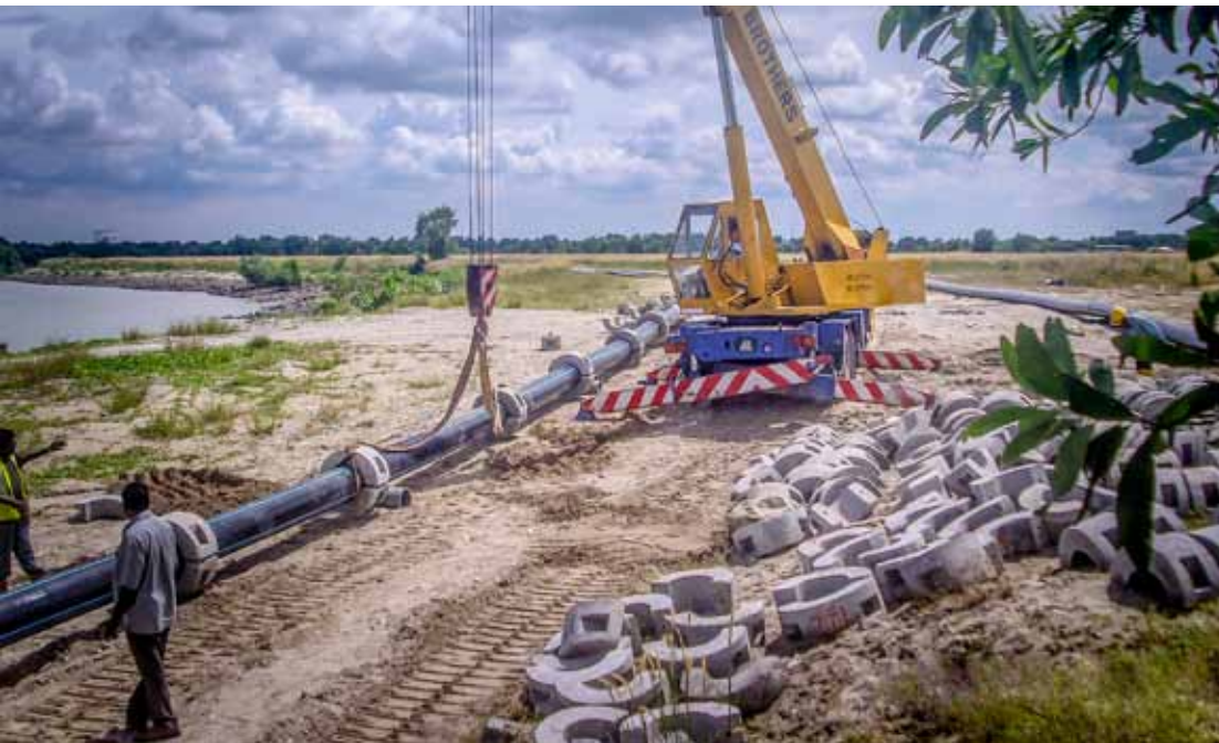
WORK // WATER DISTRIBUTION NETWORK LOCATION // PULAU INDAH
