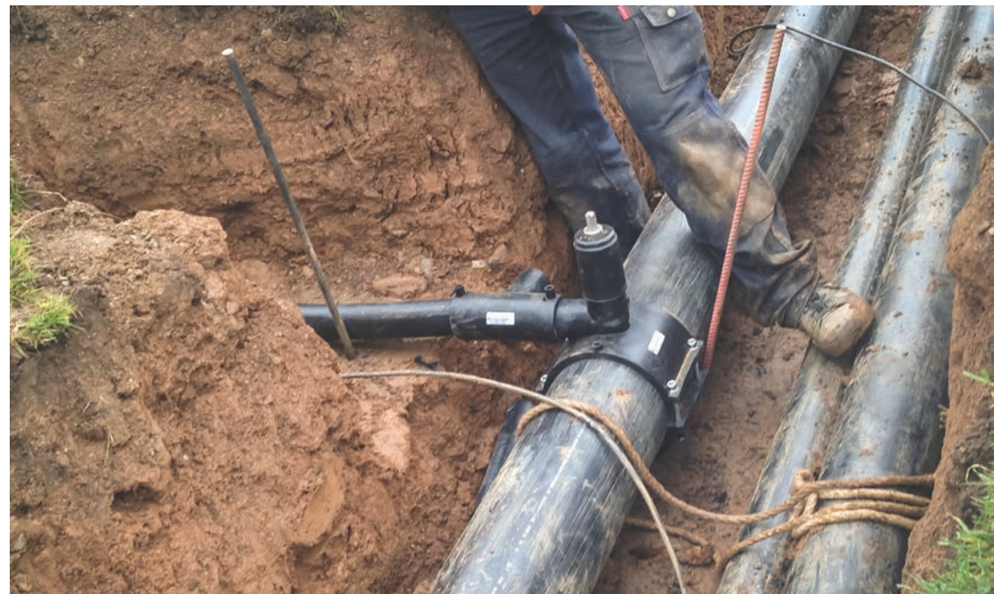
WORK // GOLF COURSE IRRIGATION PLANT LOCATION // GOLF DE VALCROS - LA LONDE-LES-MAURES
