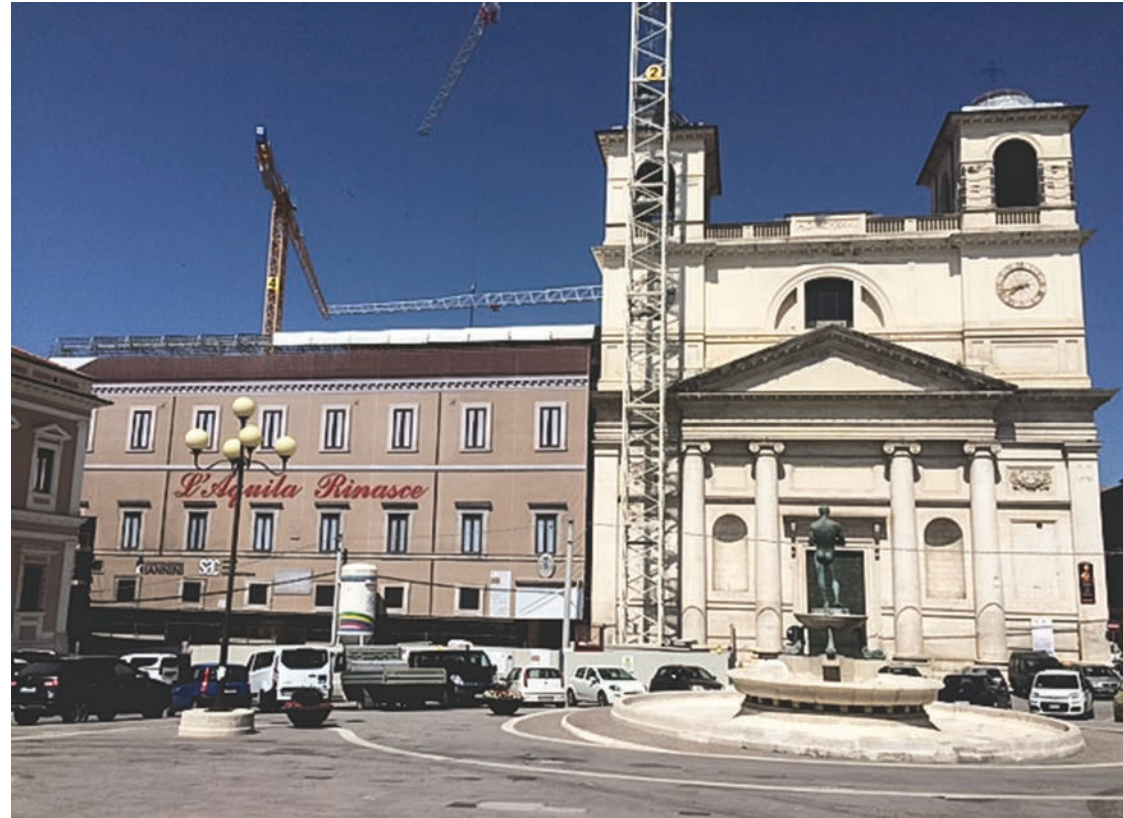
WORK // UNDERGROUND SUBSERVICES TUNNEL LOCATION // L'AQUILA
