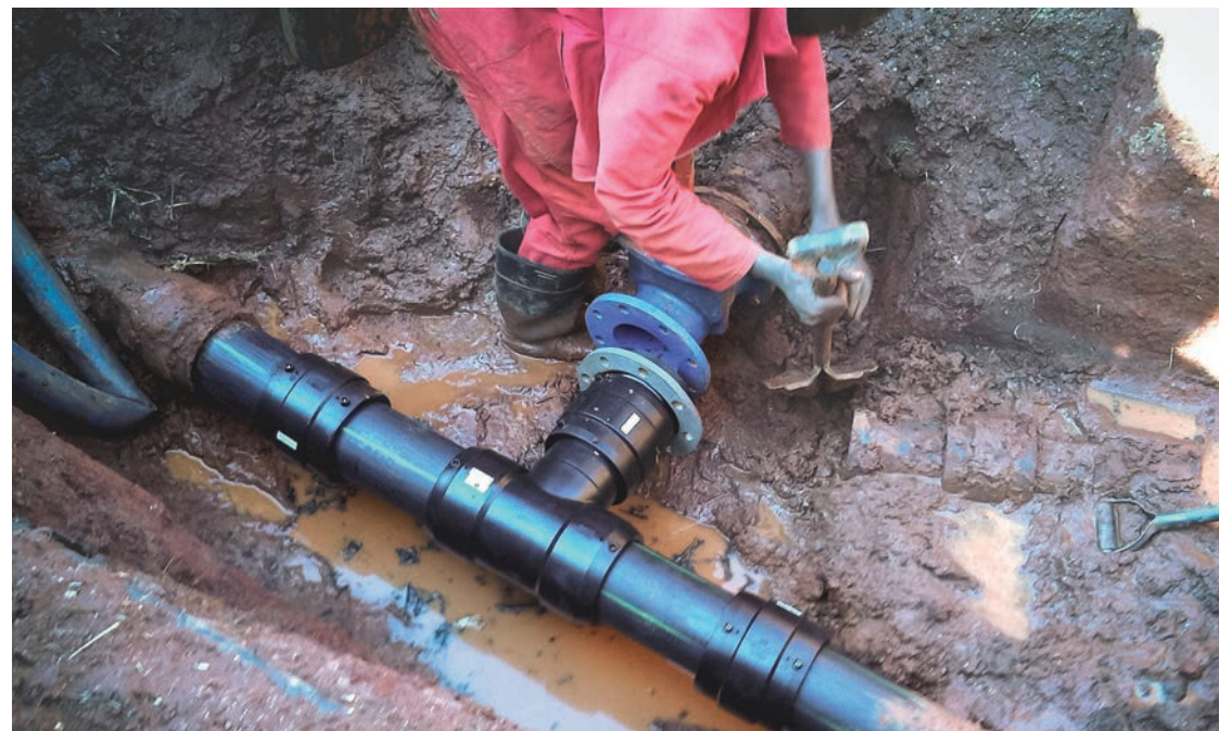
WORK // WATER DISTRIBUTION NETWORK LOCATION // NELSPRUIT – PROVINCE OF MPUMALANGA
