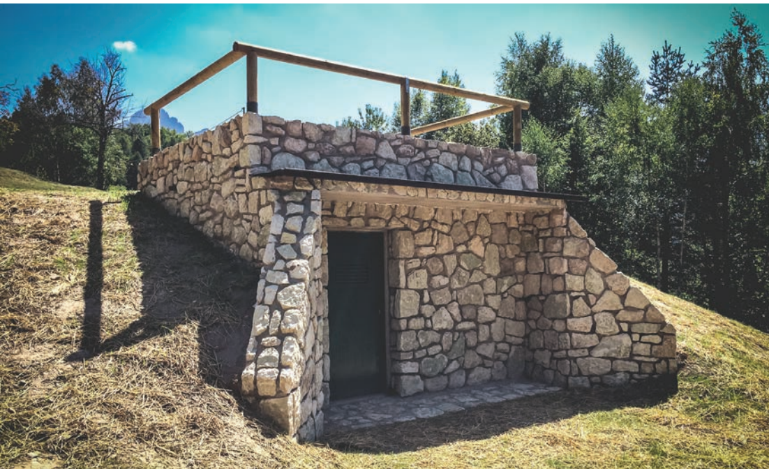
WORK // IRRIGATION PLANT DISTRIBUTION FRAME LOCATION // VALLARSA - TRENTO
