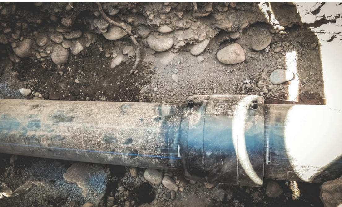
WORK // WATER DISTRIBUTION RENOVATION LOCATION // MAIPU - SANTIAGO
