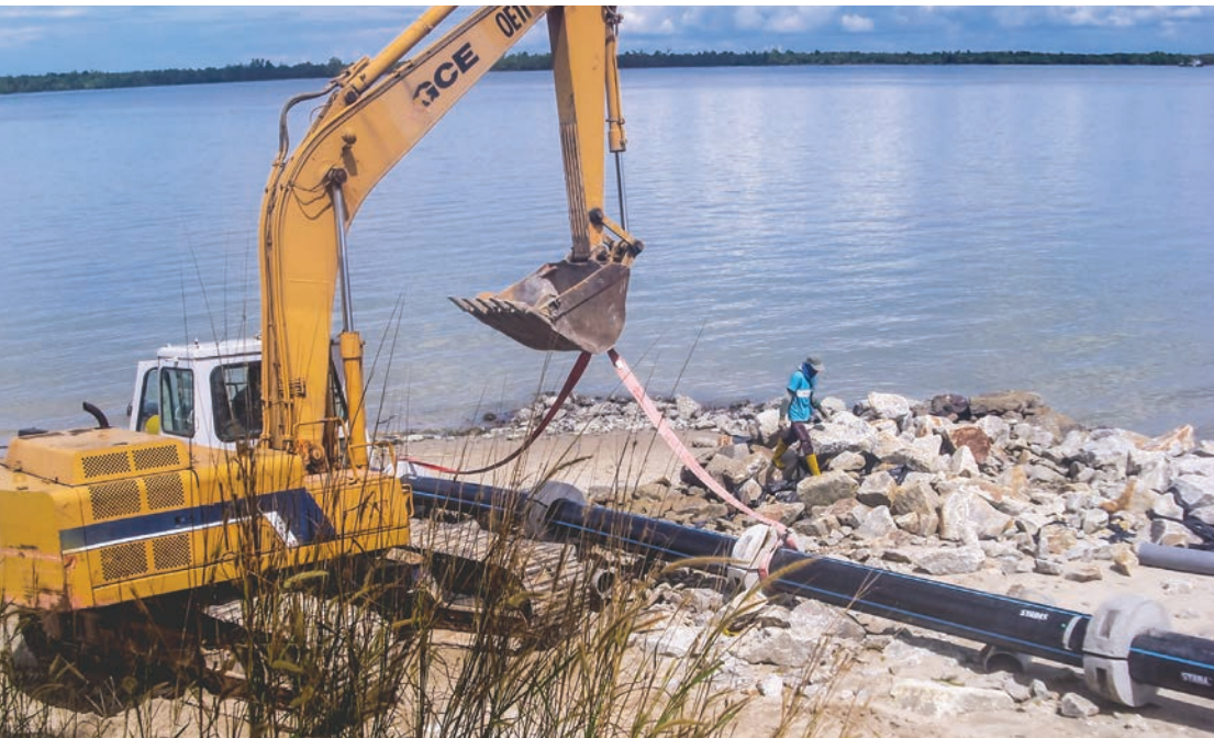
WORK // SUBMARINE WATER PIPELINE LOCATION // PULAU INDAH ISLAND - SELANGOR
