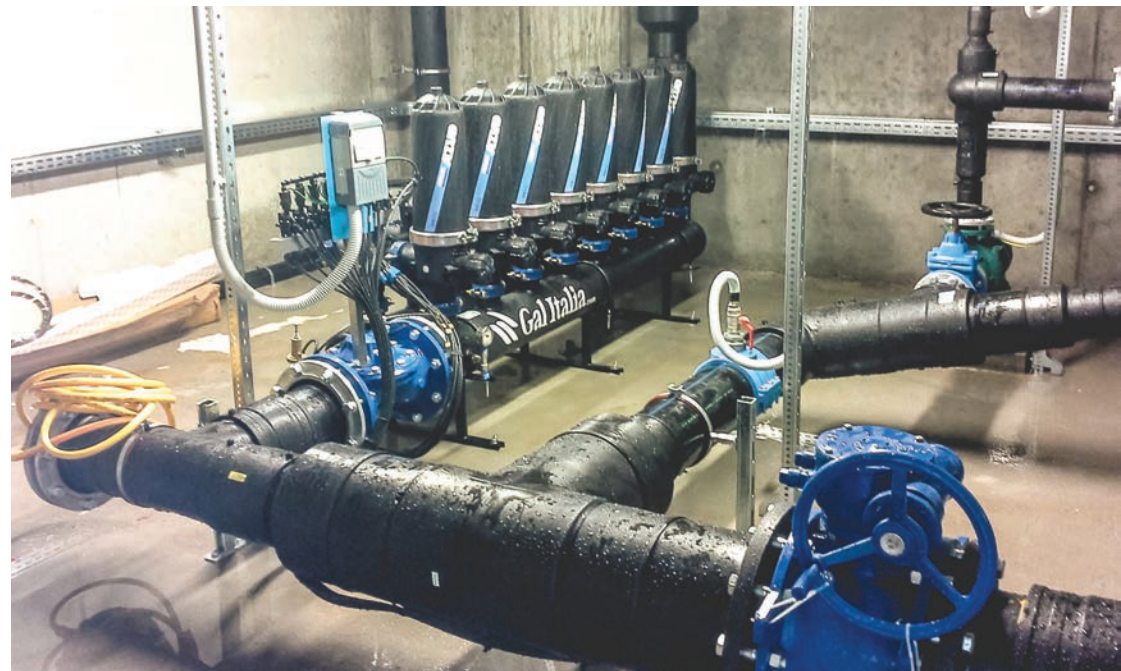
WORK // IRRIGATION FILTERING PLANT LOCATION // VILLA AGNEDO - TRENTO
