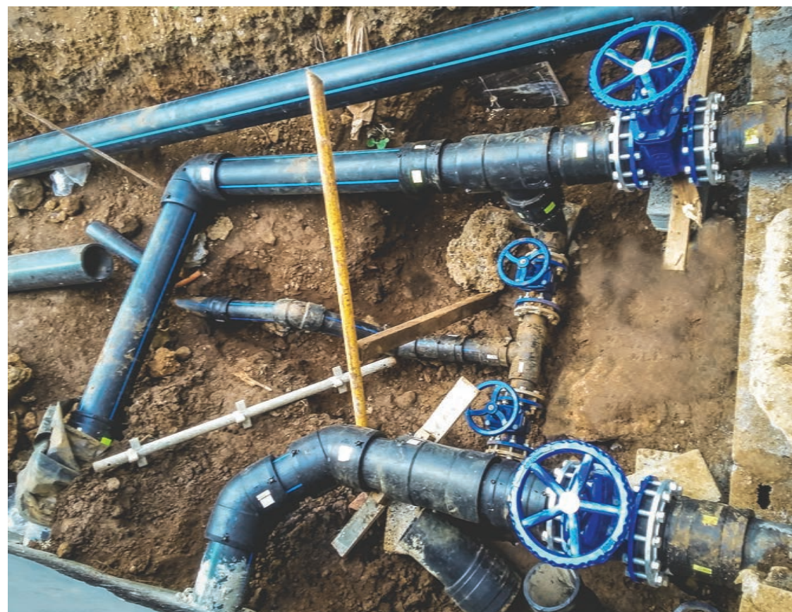
WORK // WATER PUMPING STATION LOCATION // MONT CHOISY
